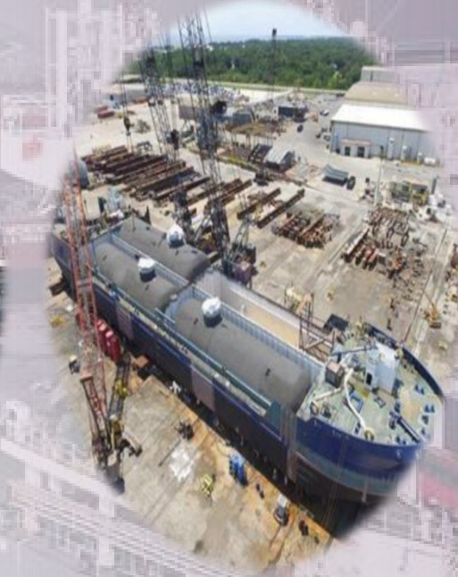
CHS (Cargo Handling System)
